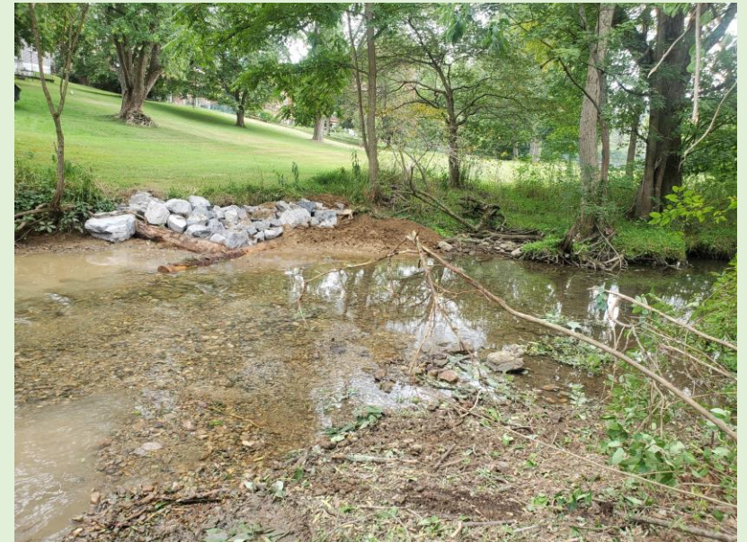
August 7 – Log-framed rock deflector adjacent to large mud-sill.
