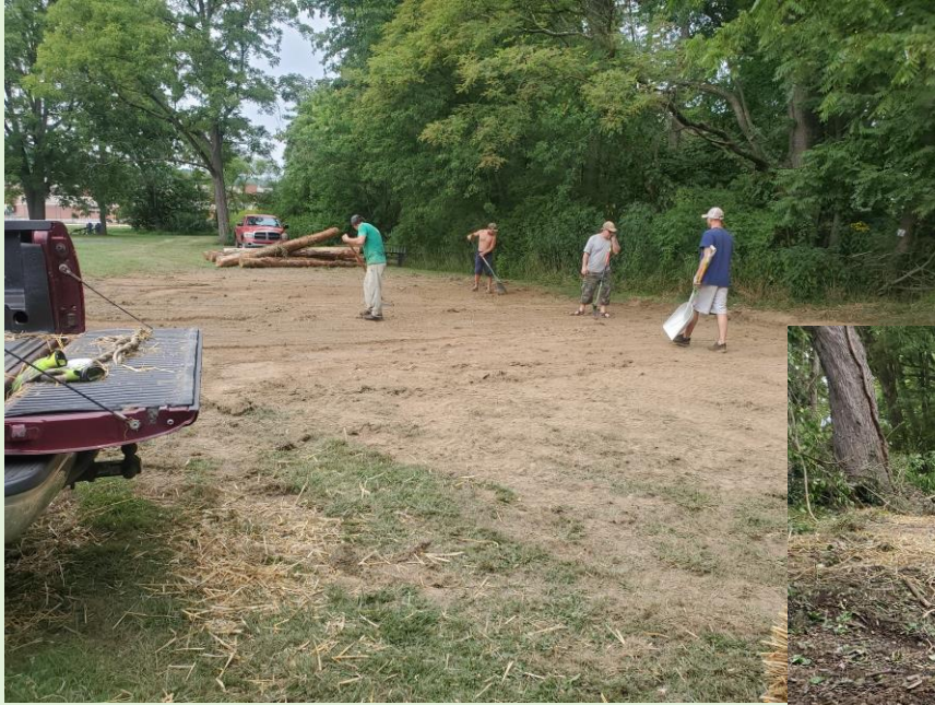
August 7, 2021 – Smoothing tire ruts and picking rocks.
